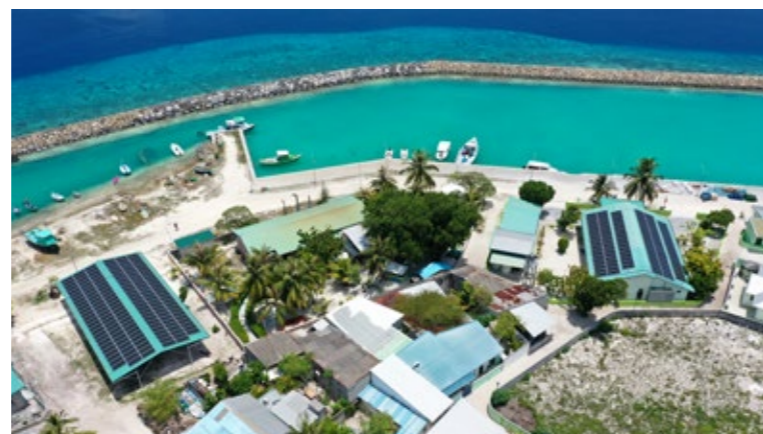
The solar power project at the Kuredu Resort & Spa, one of many Maldivian resorts now employing solar technology. Photo: Ministry of Environment and Energy
